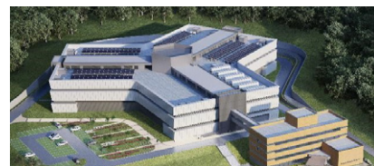
(Chuncheon DC) Photovoltaic Power Generation
