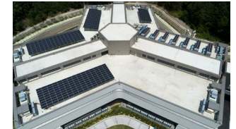
Chuncheon Data Center Solar Power Generation Facility
