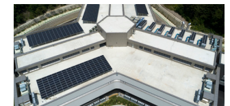
Chuncheon DC Photovoltaic Power Generation
