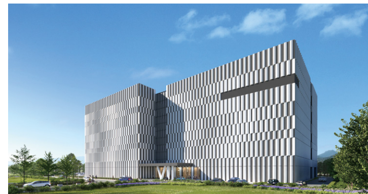
Dongtan Data Center
