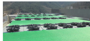
Chuncheon DC Shading Roof
