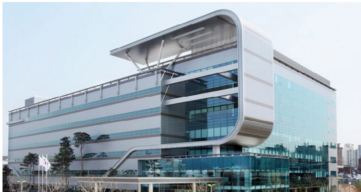
Suwon Data Center
