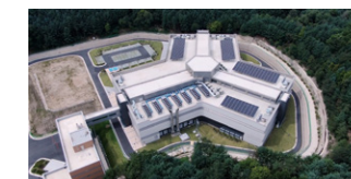
Chuncheon DC Photovoltaic Power Generation
