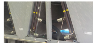
Spraying Water onto Condenser
