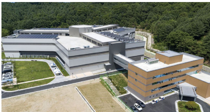
Chuncheon Data Center
