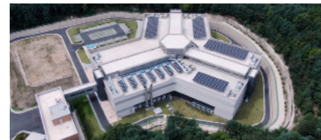
Chuncheon DC Photovoltaic Power Generation
