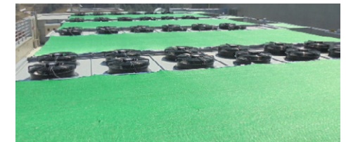
Chuncheon DC Shading Roof
